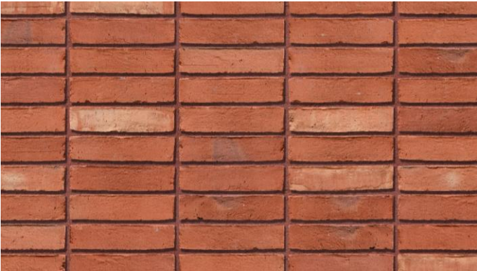
Red brick cladding
