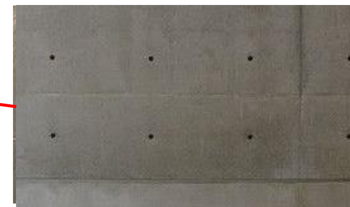
Cast in place Concrete landscape walls
