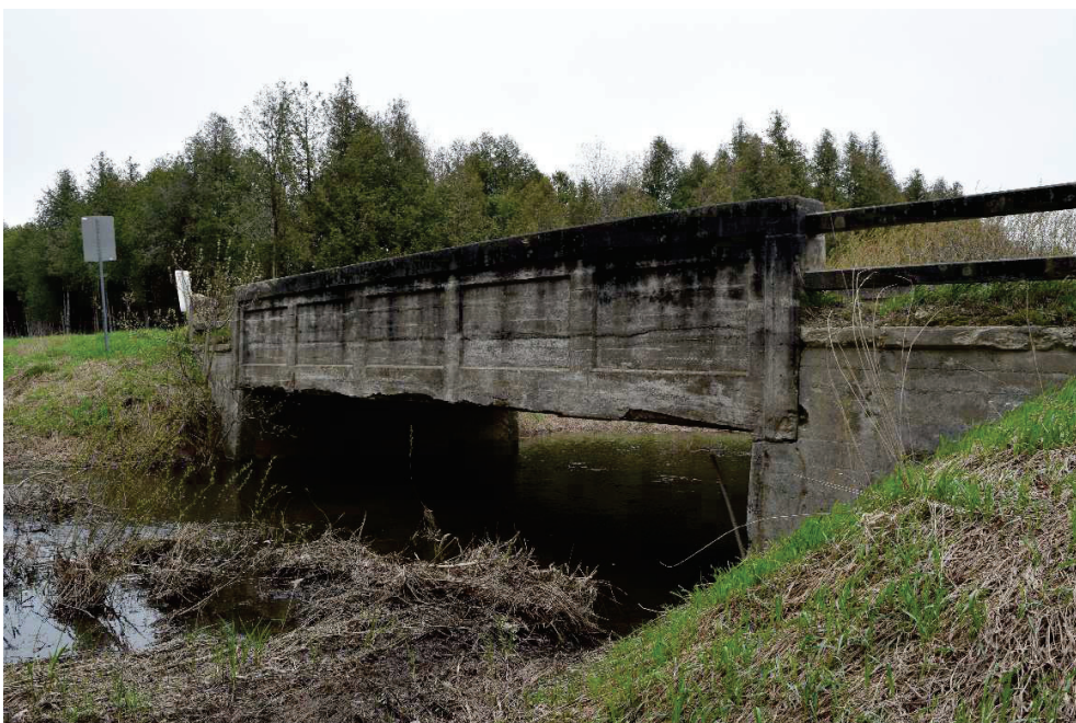
IMAGE 2: 2-WG WITH STEEP DITCHES, FACING SOUTH
