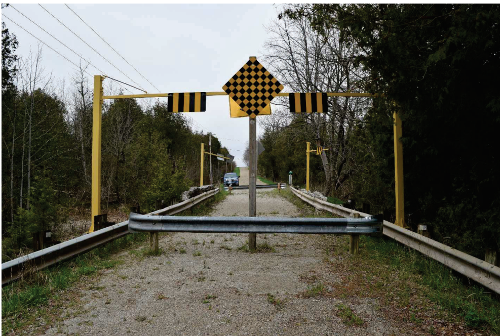
IMAGE 14: 7-E WITH STEEP DITCHES TO POORLY DRAINED ENVIRONS, FACING NORTHWEST
