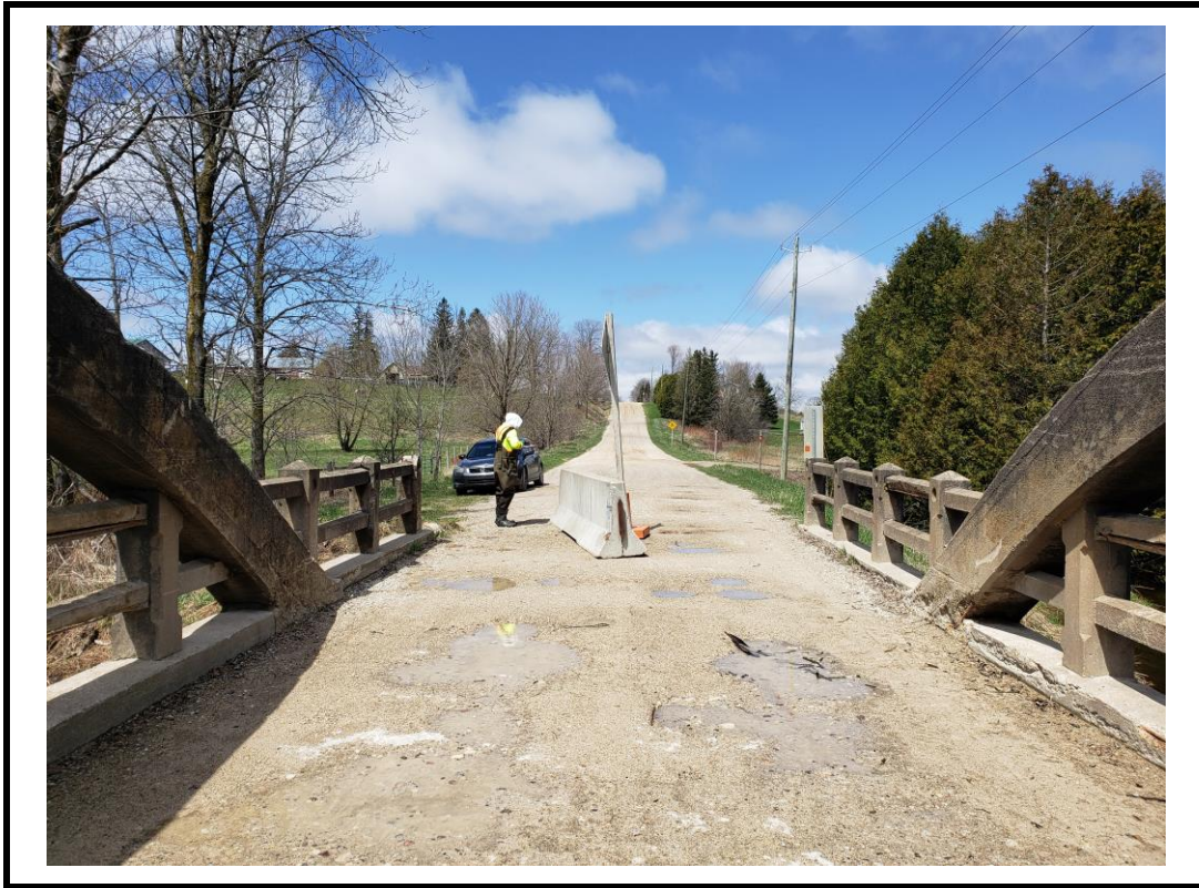
Photo 3 North approach from centre of structure
