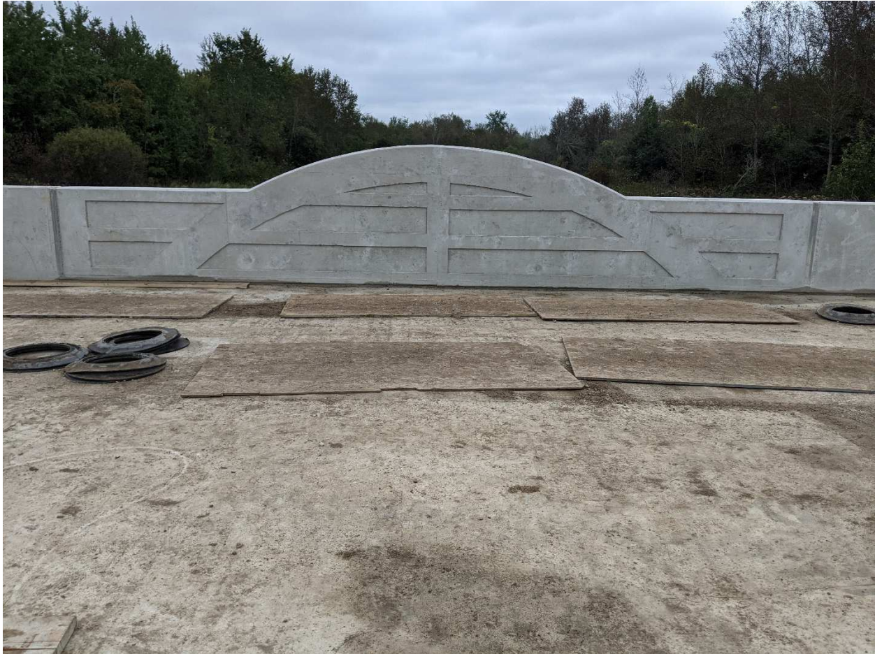
FIGURE 10: BRIDGE 4-F, TOWNSHIP OF CENTRE WELLINGTON
