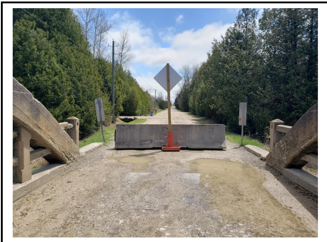
Photo 4 South approach from centre of structure
