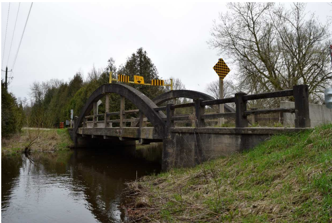
FIGURE 3: BRIDGE 3-E, SOUTHSIDE OF BRIDGE, FACING NORTH
