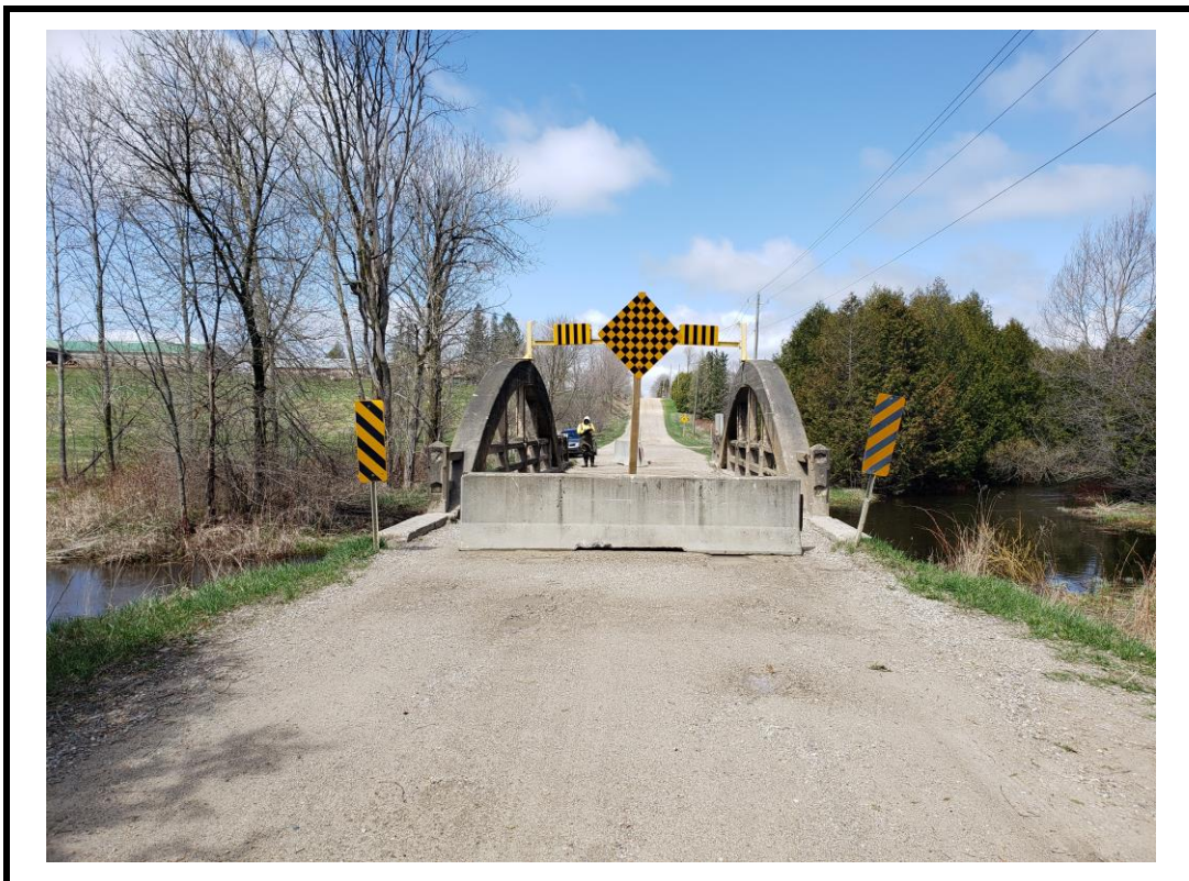
Photo 2 Structure from south approach
