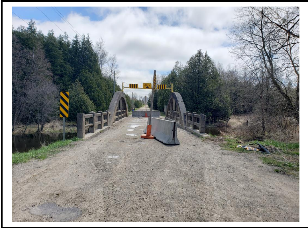
Photo 1 Structure from north approach
