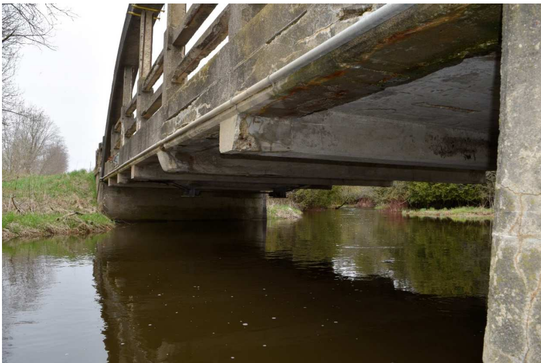
FIGURE 8: BRIDGE 3-E, UNDERSIDE OF BRIDGE DECK
