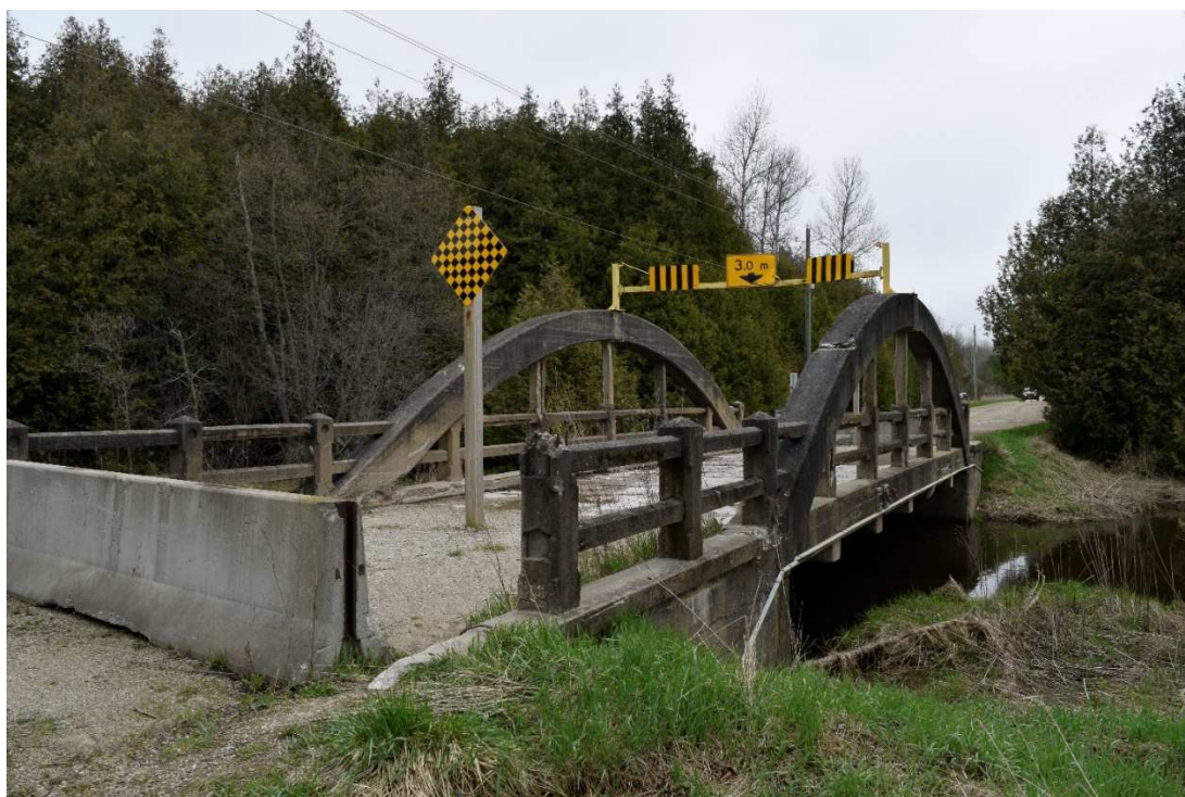
FIGURE 2: BRIDGE 3-E, SOUTH SIDE OF BRIDGE, FACING NORTH
