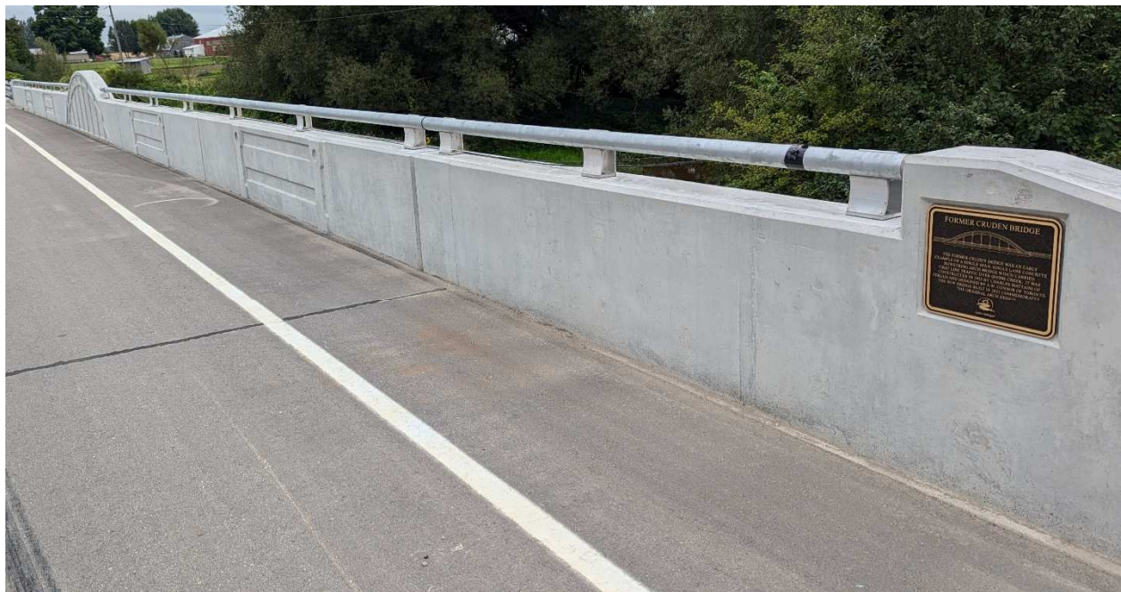
FIGURE 9: BRIDGE 24-WG, TOWNSHIP OF CENTRE WELLINGTON
