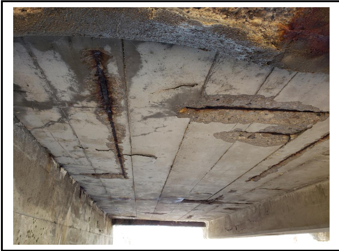
Photo 11 Spalls with exposed corroded rebar and delamination at soffit
