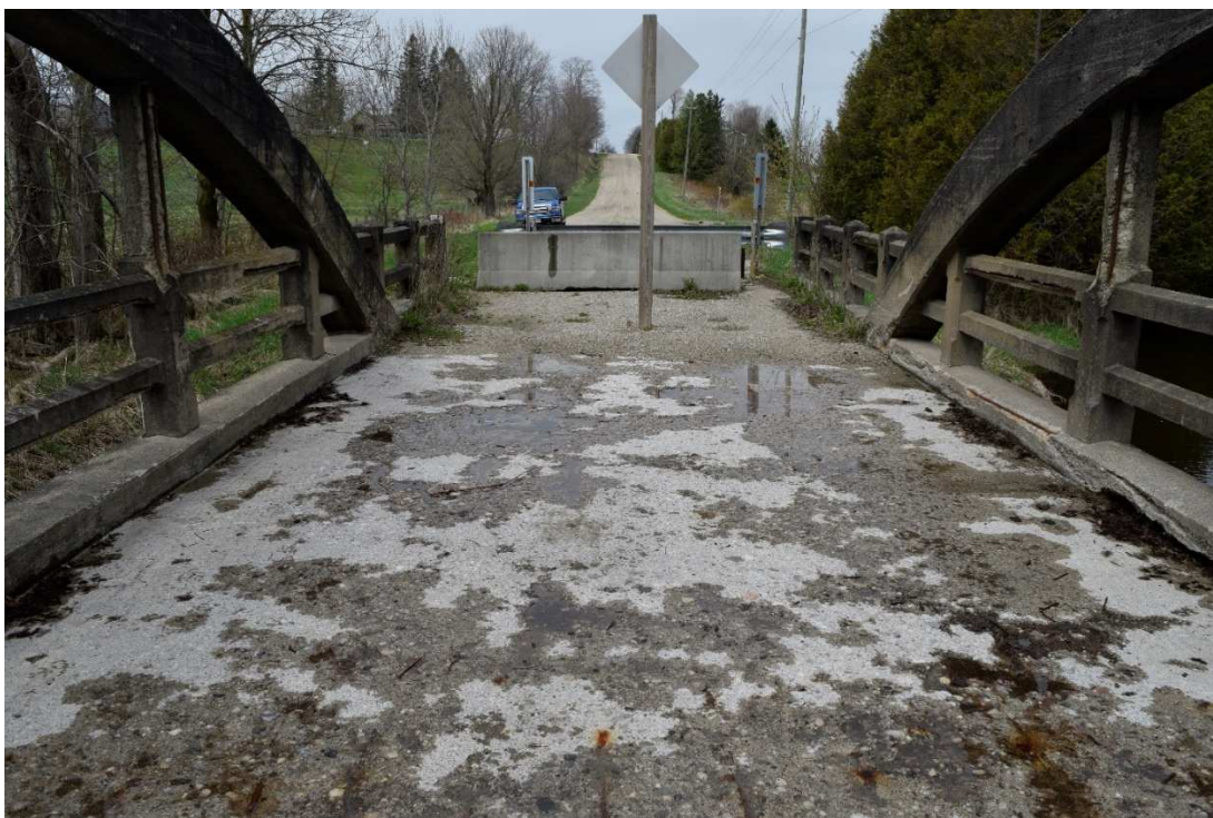
FIGURE 6: BRIDGE 3-E, BRIDGE DECK, FACING NORTHWEST
