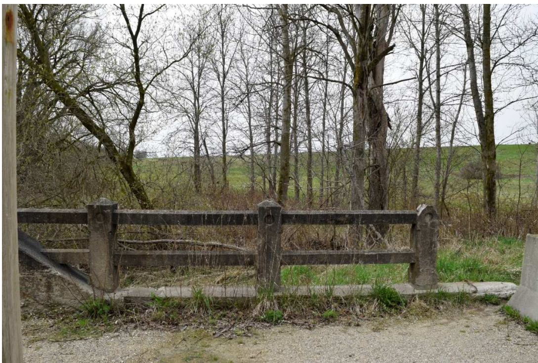
FIGURE 4: BRIDGE 3-E, TYPICAL GUARDRAIL, SOUTH SIDE
