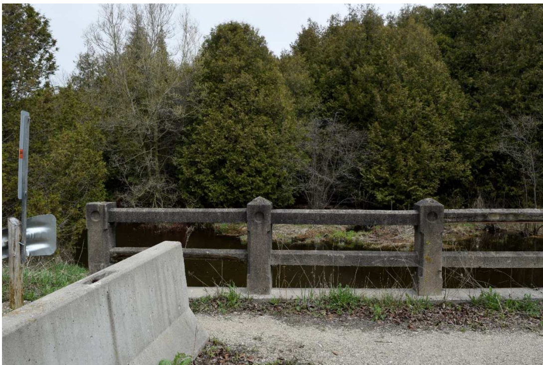
FIGURE 5: BRIDGE 3-E, TYPICAL GUARDRAIL NORTH SIDE
