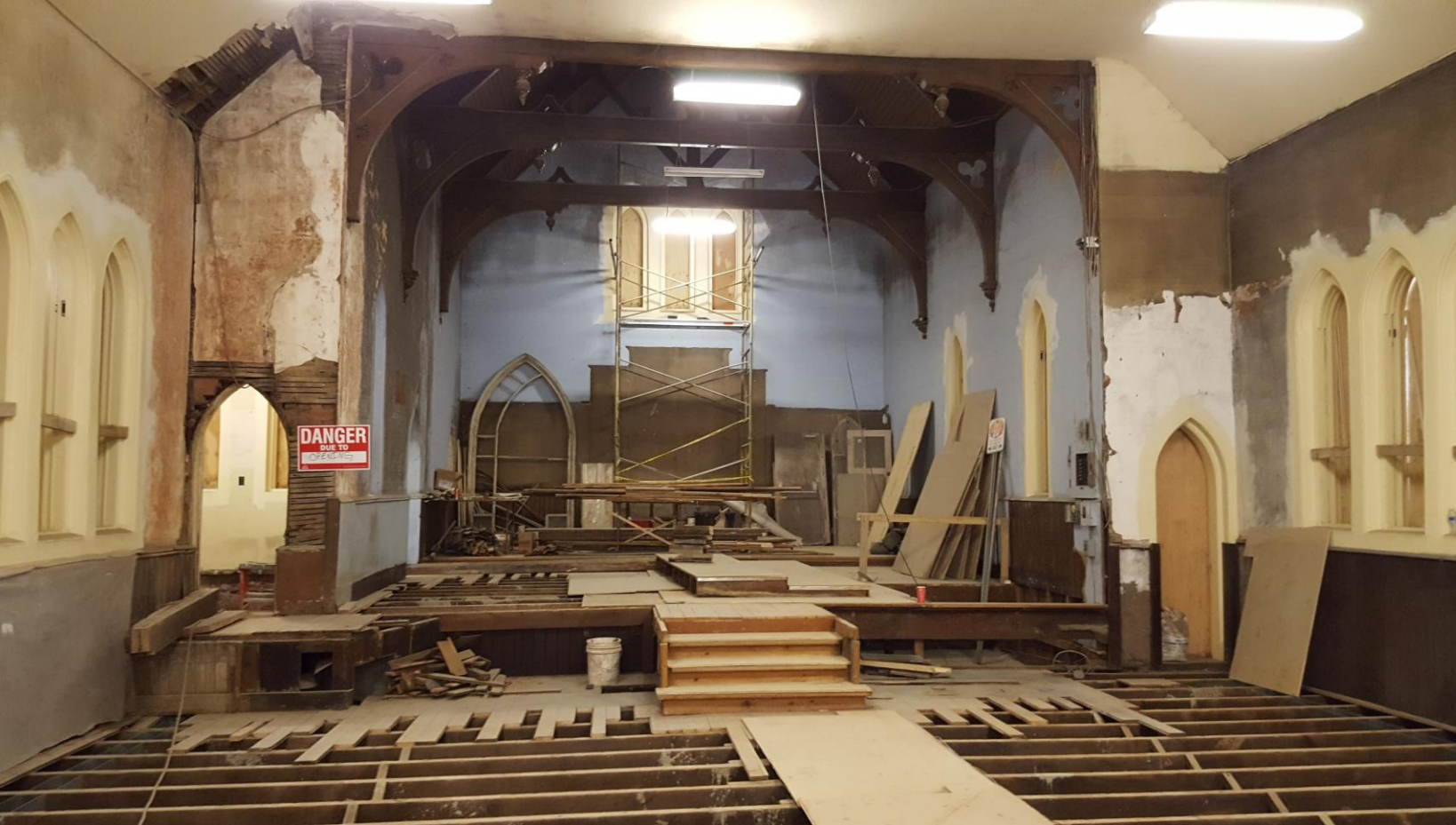
St Marks / Magnolia Hall – City of Hamilton
