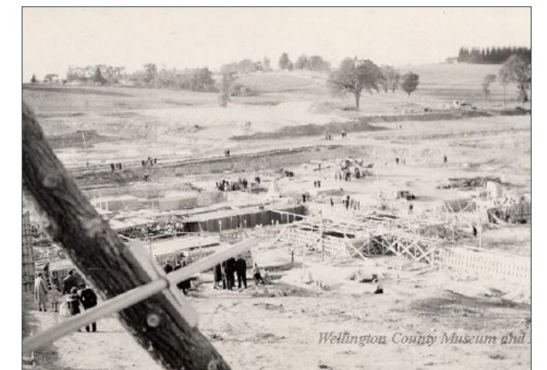
Shand Dam under construction, 1939 (W.C.M.A. Ph10785).
