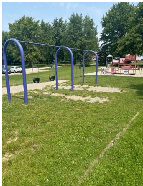
Pictured above: Strathallan Park, general wear present in playground structure.
