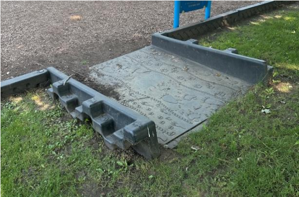
Pictured above: example of an accessible curb ramp / opening, Drimmie Park.
