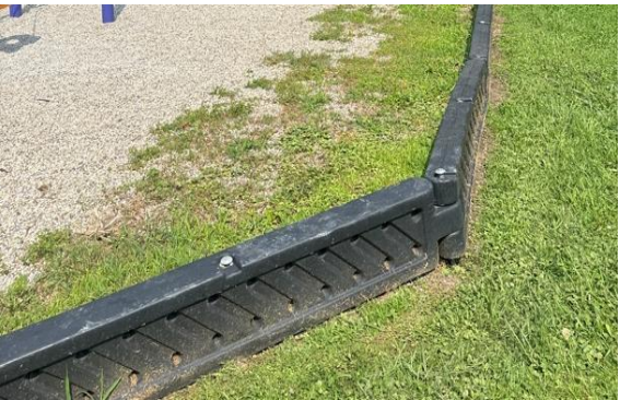
Pictured above: examples of playground raised curbs at Strathallan Park (top) and Wilkie Park (bottom)
