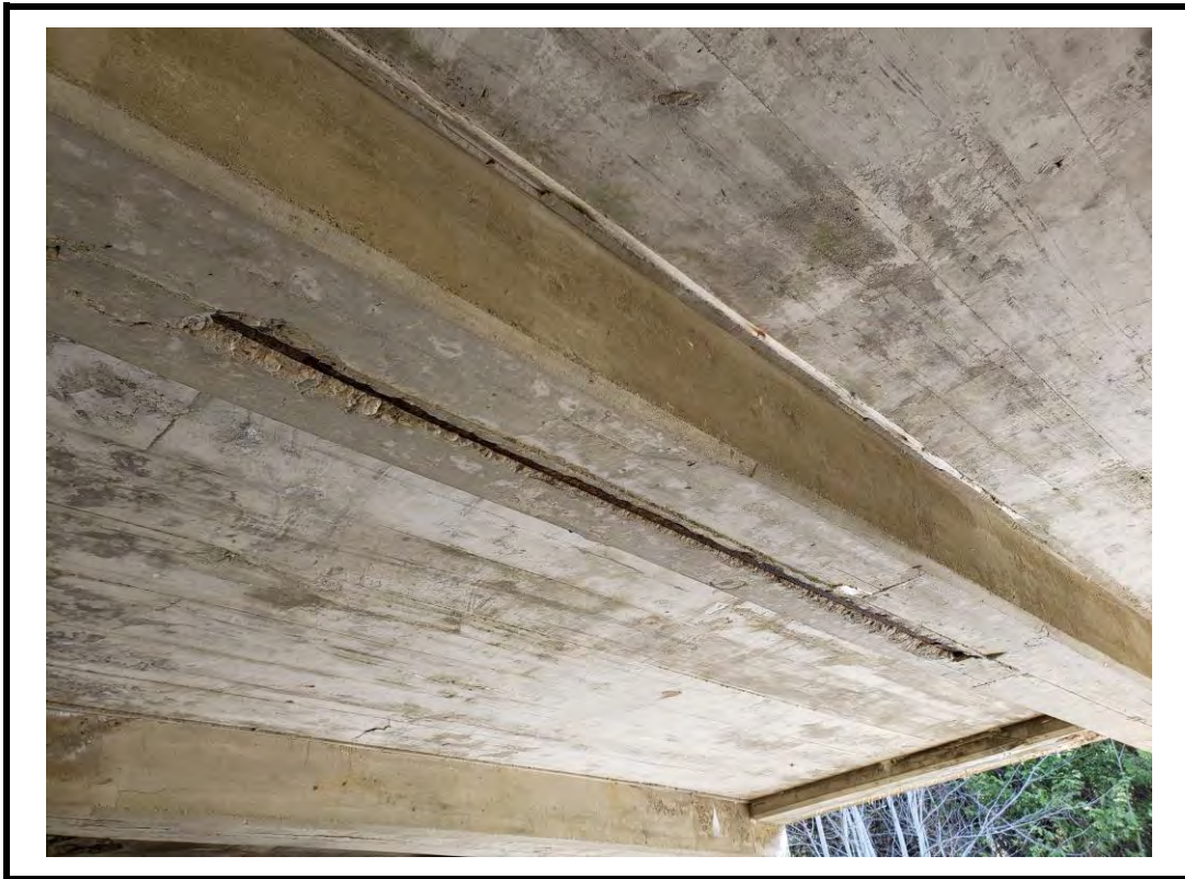
Photo 11 Spall with exposed corroded reinforcing and efflorescence on girder & floor beam
