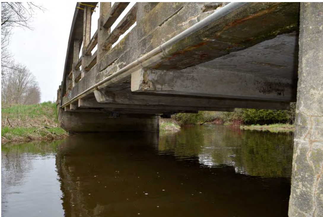
FIGURE 17: BRIDGE 3-E, UNDERSIDE OF BRIDGE DECK
