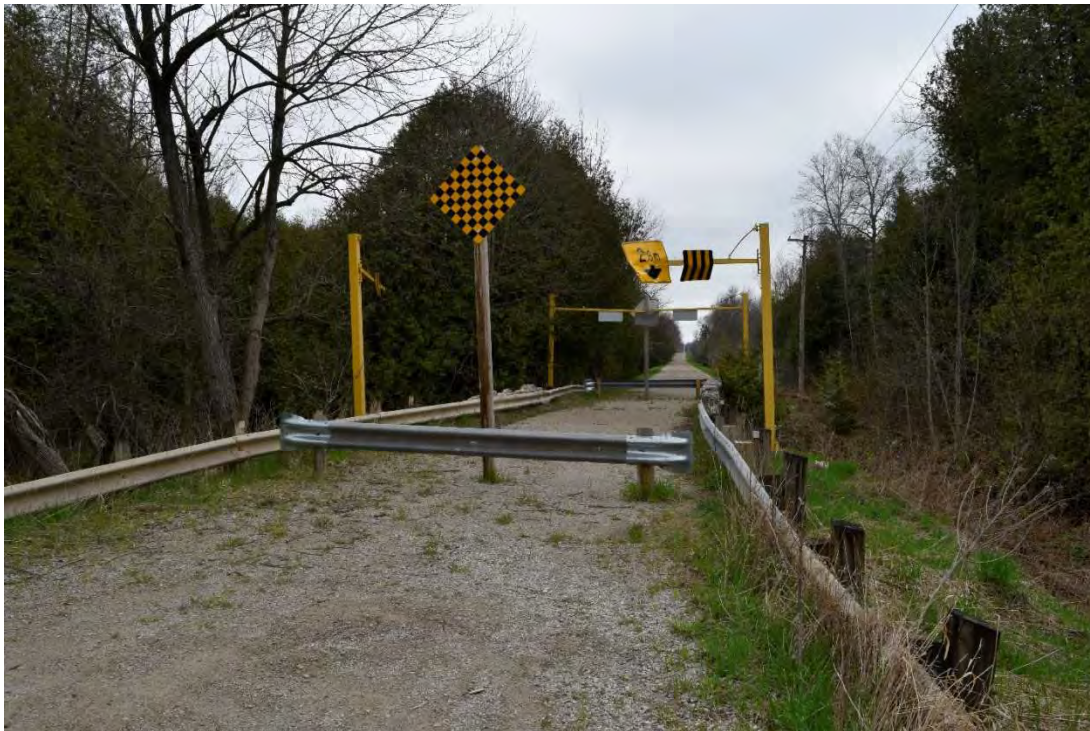
FIGURE 24: BRIDGE 7-E, NORTH APPROACH TO BRIDGE, FACING SOUTH
