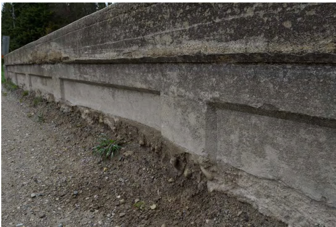
FIGURE 5: BRIDGE 2-WG, CLOSE UP OF SUPERSTRUCTURE
