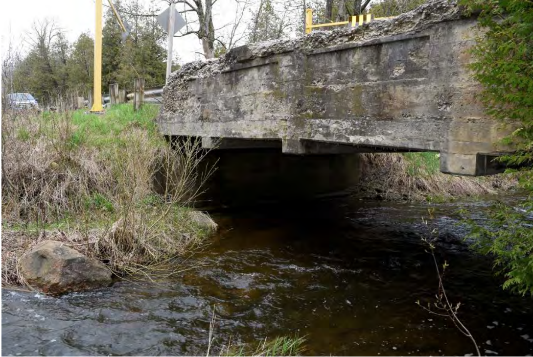
FIGURE 27: BRIDGE 7-E, OVERVIEW OF THE WEST SIDE OF BRIDGE, FACING NORTH
