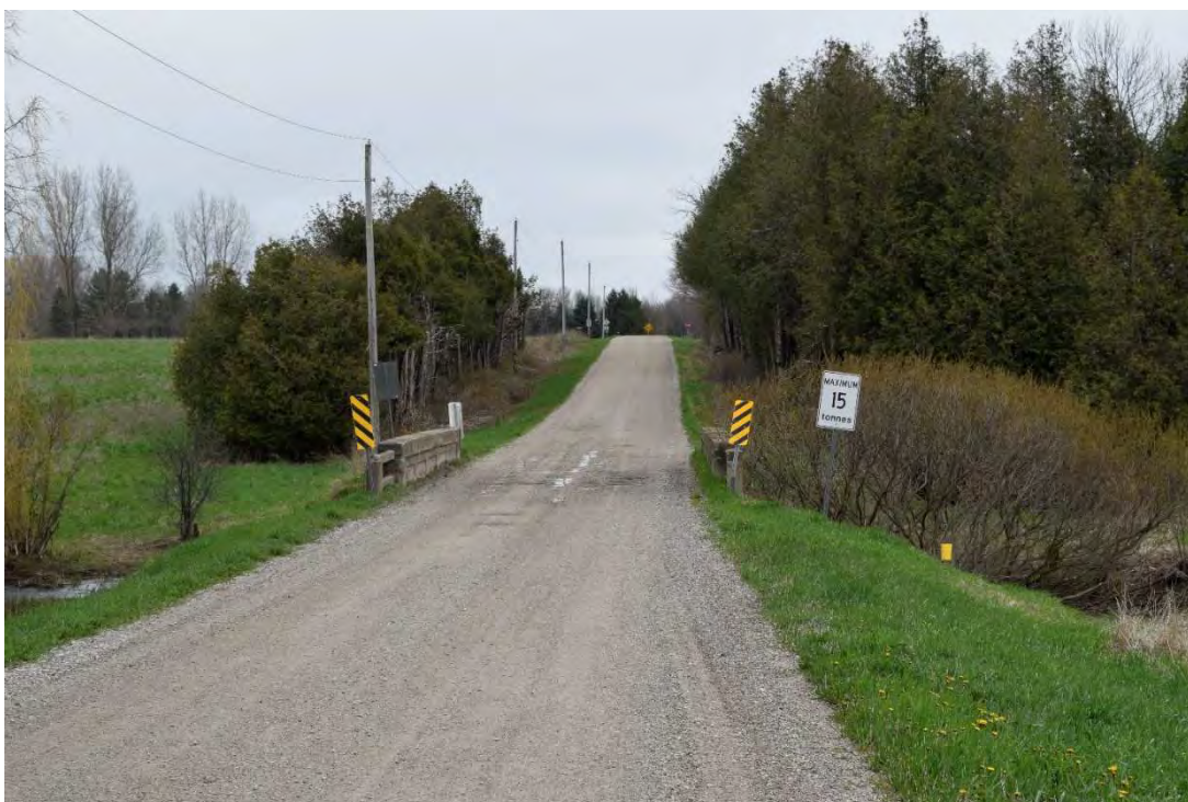
FIGURE 9: BRIDGE 2-WG, APPROACH TO BRIDGE 2-WG FACING SOUTHEAST
