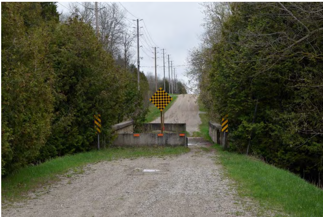
FIGURE 18: BRIDGE 5-E, LOOKING SOUTHEAST FROM APPROACH
