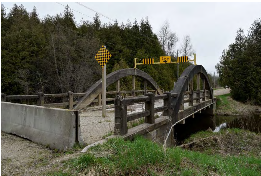
FIGURE 11: BRIDGE 3-E, SOUTH SIDE OF BRIDGE, FACING NORTH
