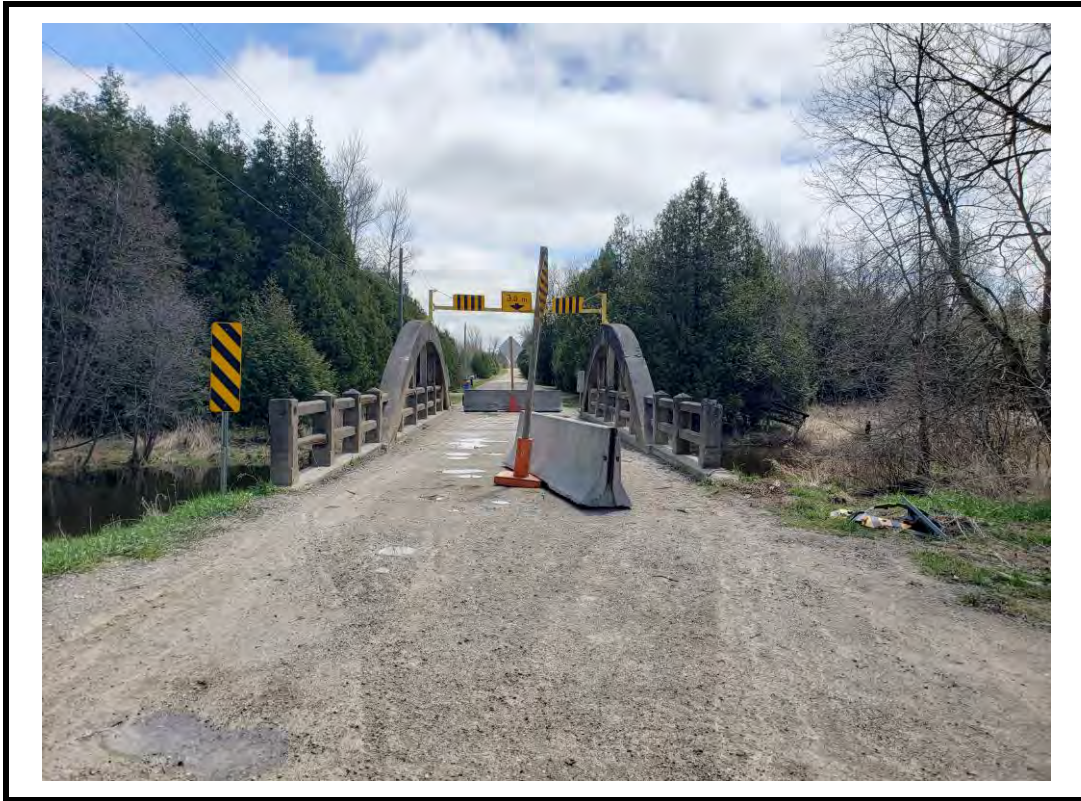
Photo 1 Structure from north approach
