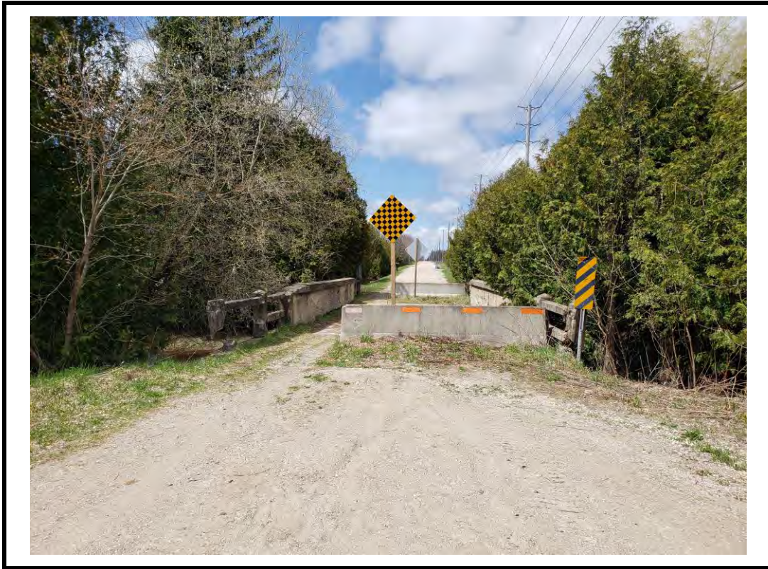
Photo 1 Structure from north approach
