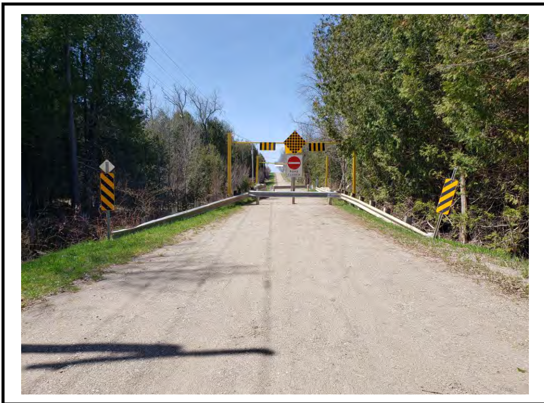
Photo 2 Structure from south approach
