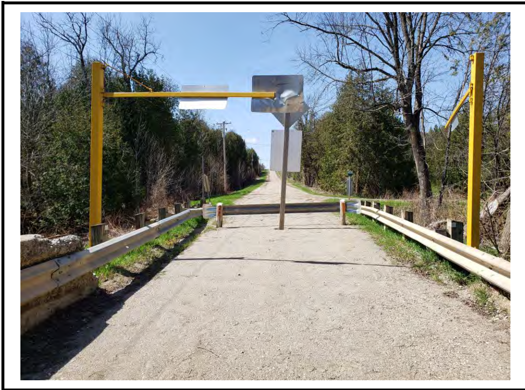
Photo 3 North approach from centre of structure
