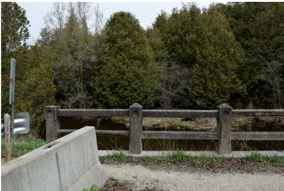
FIGURE 14: BRIDGE 3-E, TYPICAL GUARDRAIL NORTH SIDE
