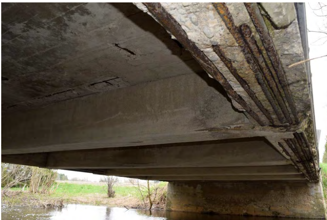
FIGURE 8: BRIDGE 2-WG, UNDERSIDE OF BRIDGE
