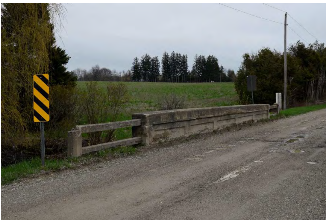
FIGURE 3: BRIDGE 2-WG, SUPERSTRUCTURE ABUTTING ROADWAY
