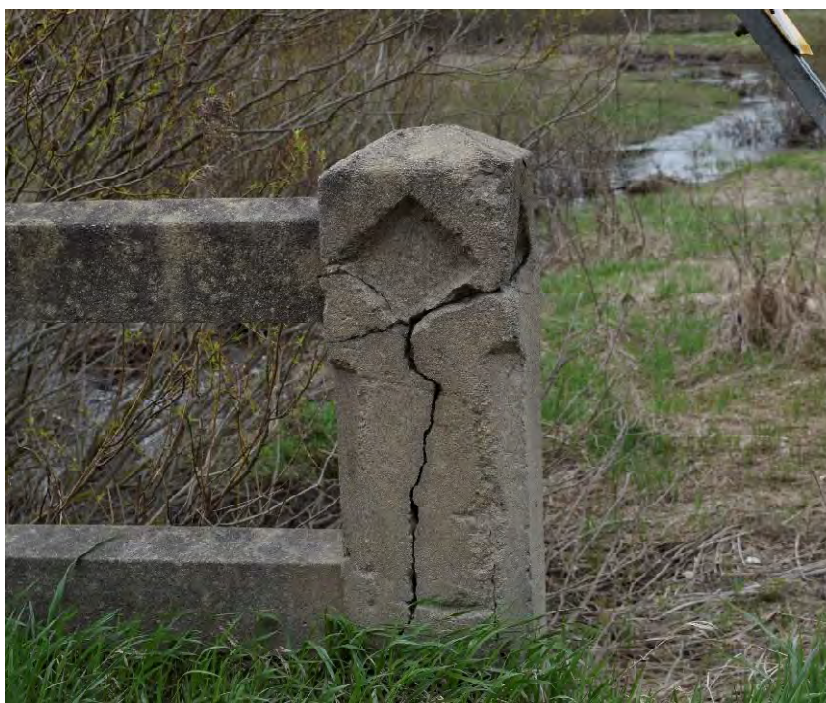
FIGURE 7: BRIDGE 2-WG, CLOSEUP OF GUARD RAIL SUPPORT WITH CHAMFERED CORNERS, CAST DIAMOND INSET AND TAPERED UPPER SURFACE
