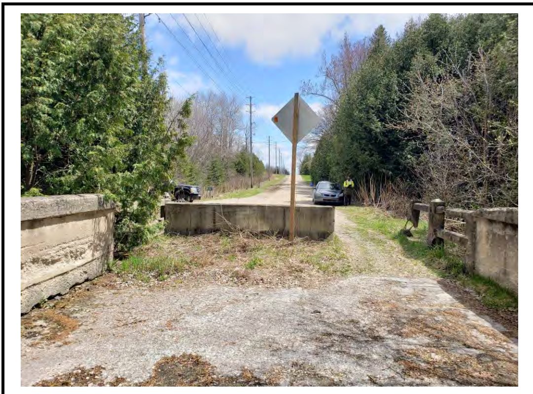
Photo 4 South approach from centre of structure
