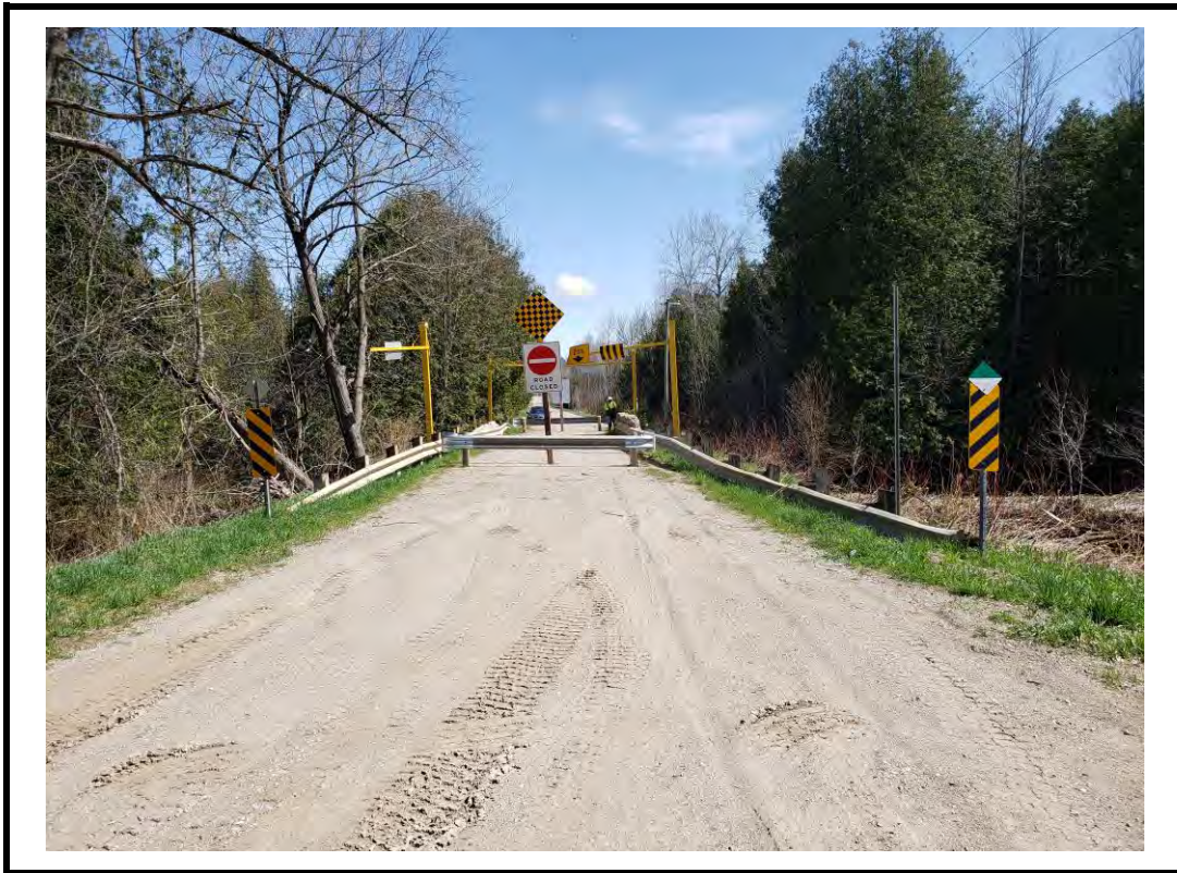
Photo 1 Structure from north approach
