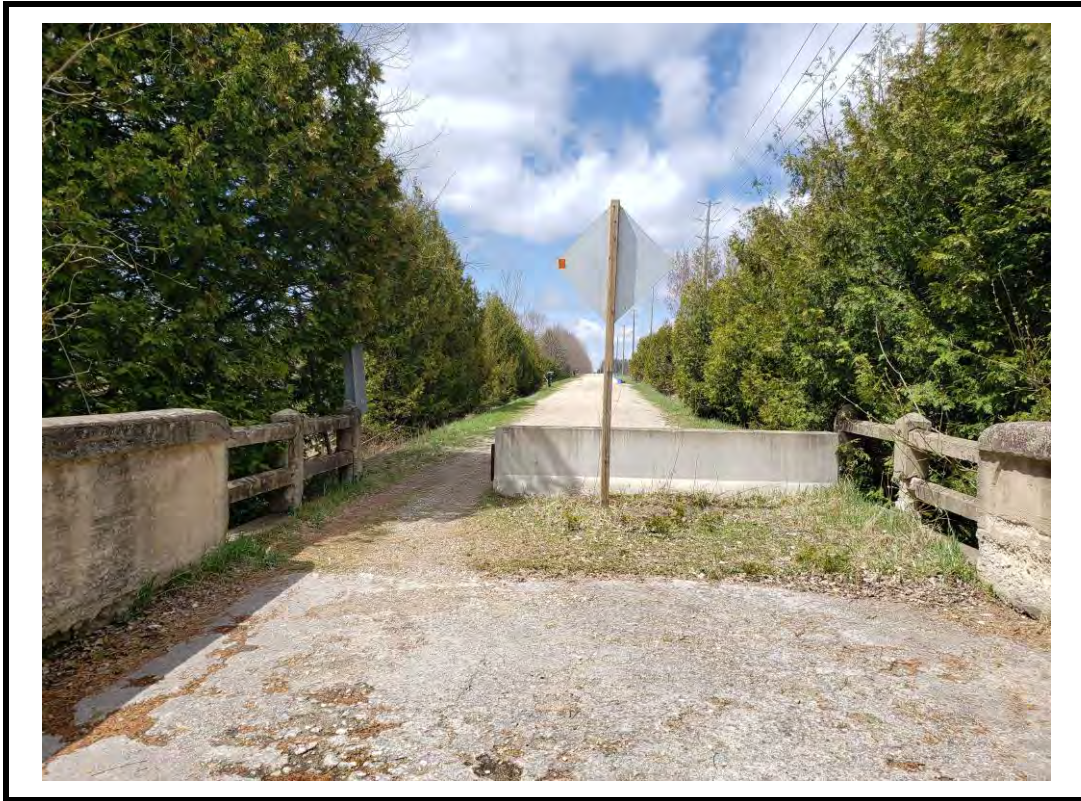
Photo 3 North approach from centre of structure
