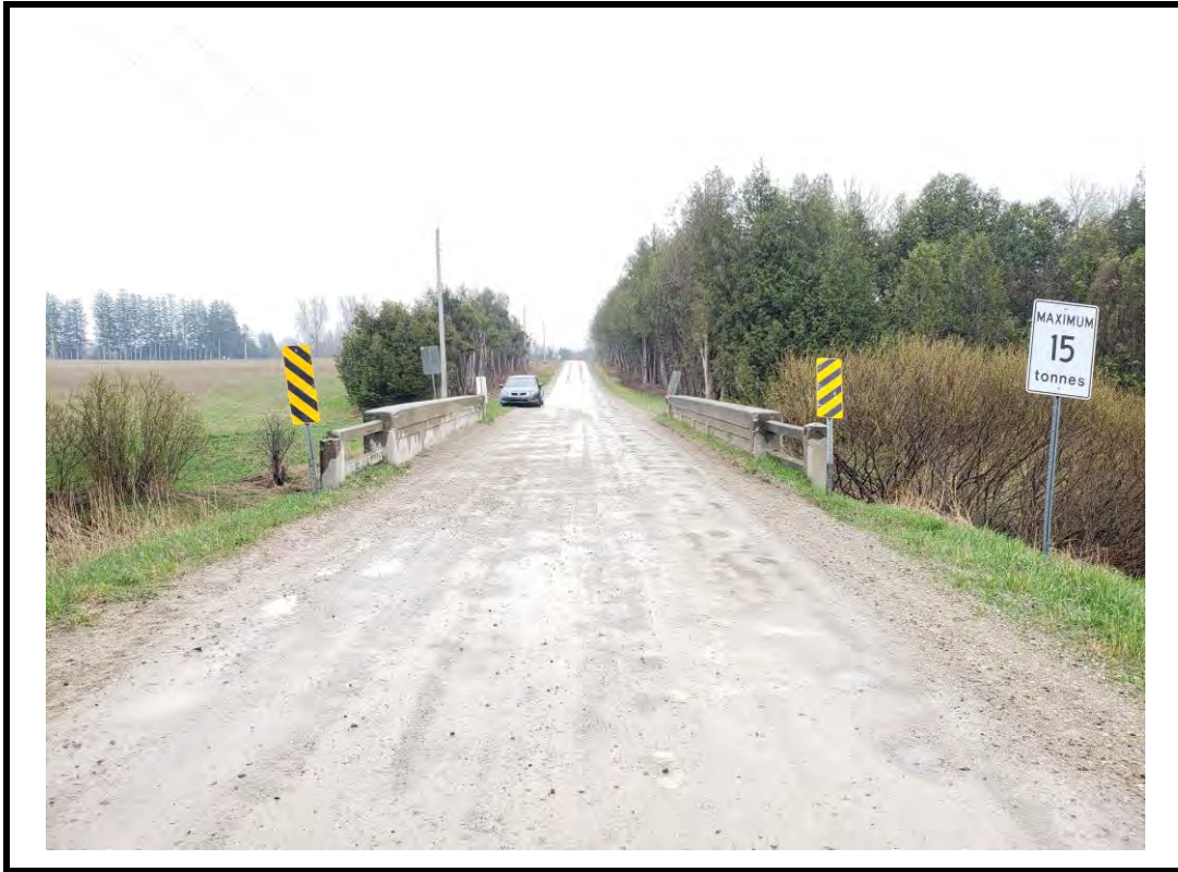
Photo 1 Structure from north approach
