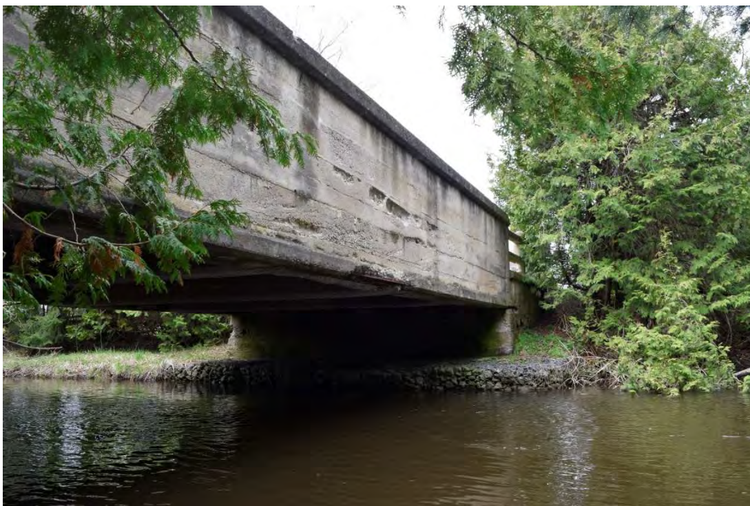
FIGURE 20: EAST SIDE OF BRIDGE 5-E
