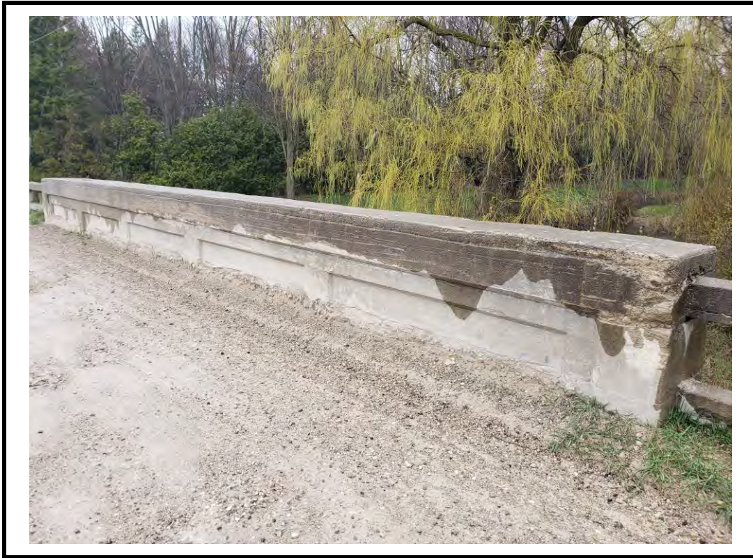
Photo 9 Interior face of west parapet wall
