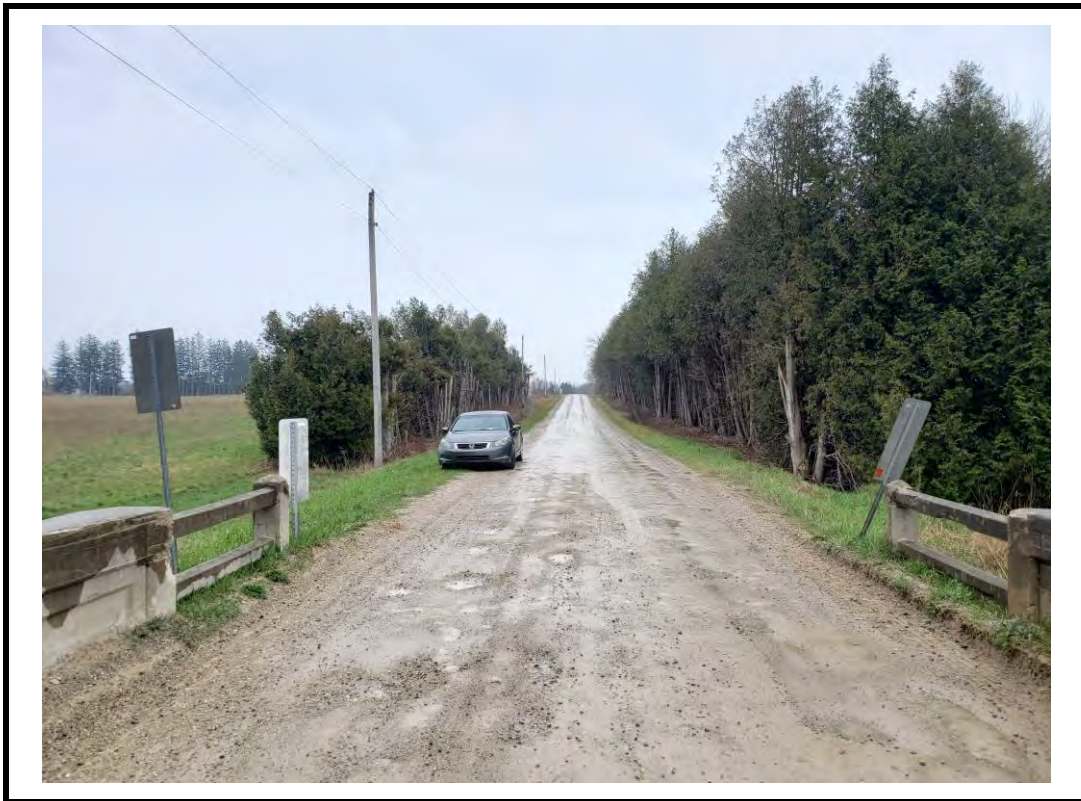
Photo 4 South approach from centre of structure
