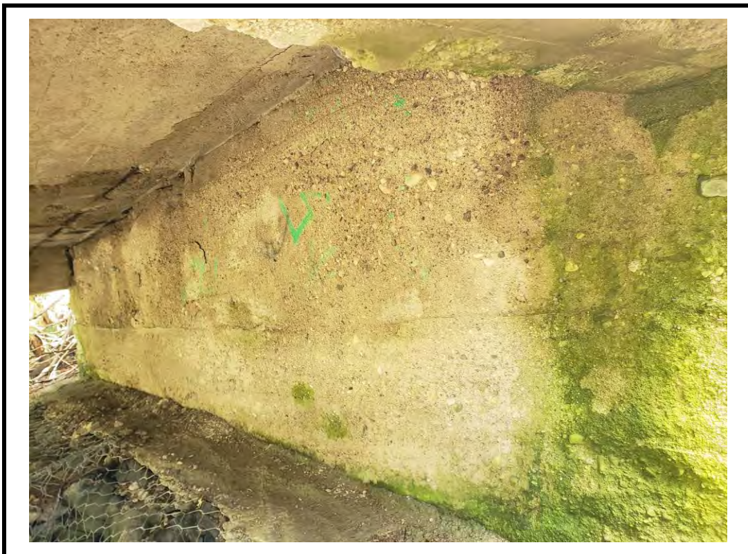
Photo 14 South abutment wall
