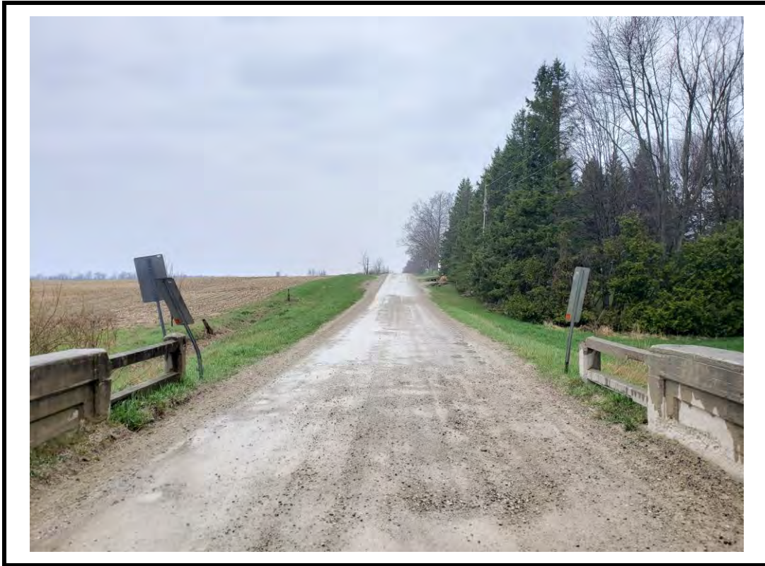
Photo 3 North approach from centre of structure
