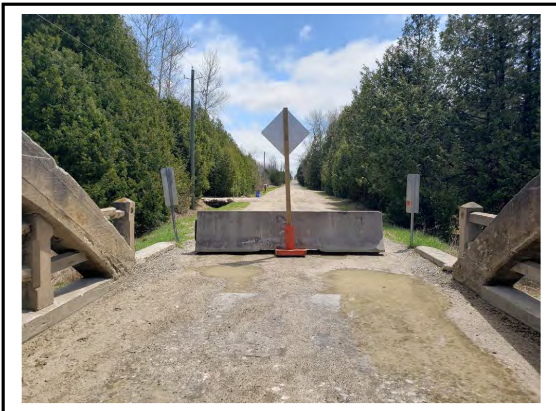
Photo 4 South approach from centre of structure
