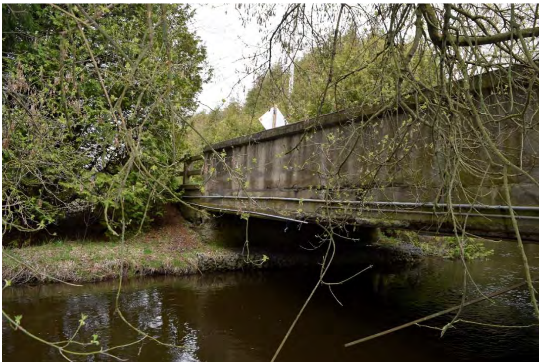
FIGURE 21: WEST SIDE OF BRIDGE 5-E
