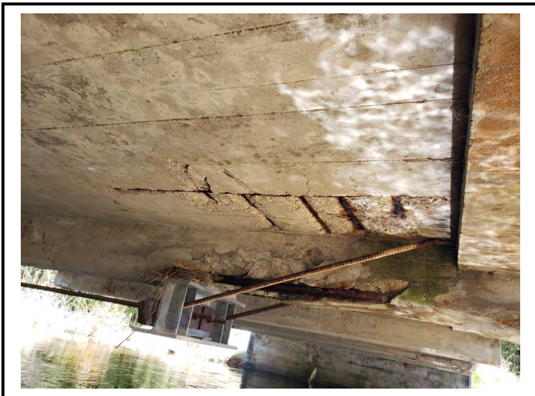
Photo 12 Large spalls with exposed corroder reinforcement at underside of floor beams and post tensioning system
