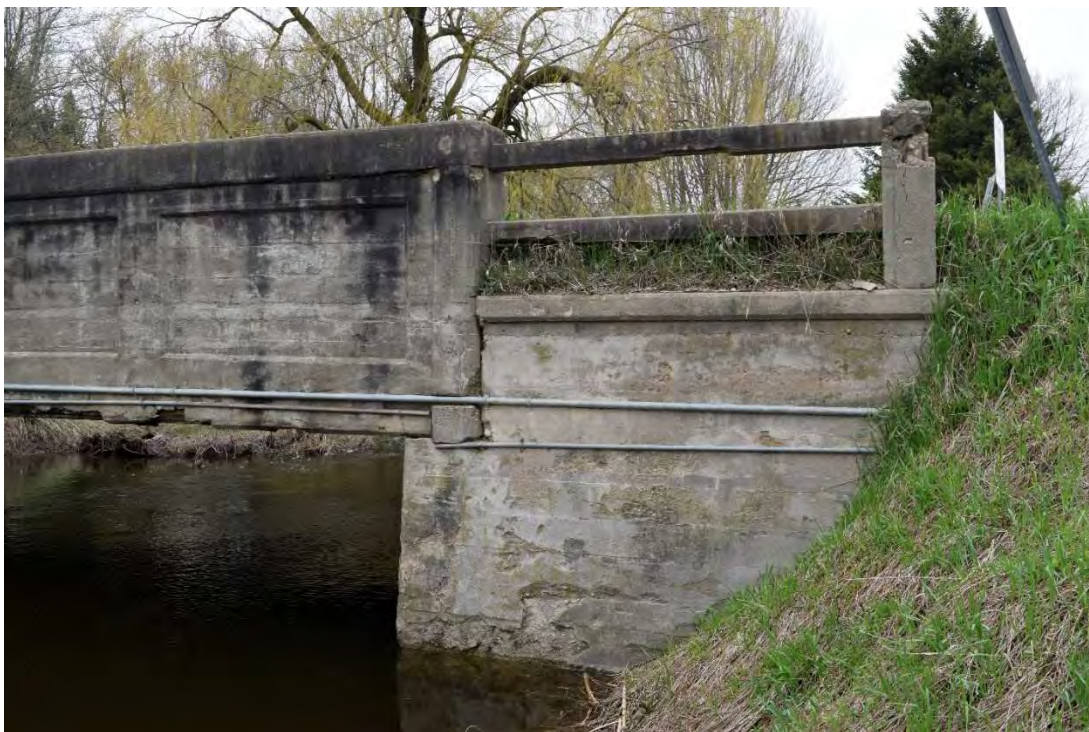
FIGURE 4: BRIDGE 2-WG, REPRESENTATIVE ABUTMENT, BRIDGE DECK AND GUARDRAIL
