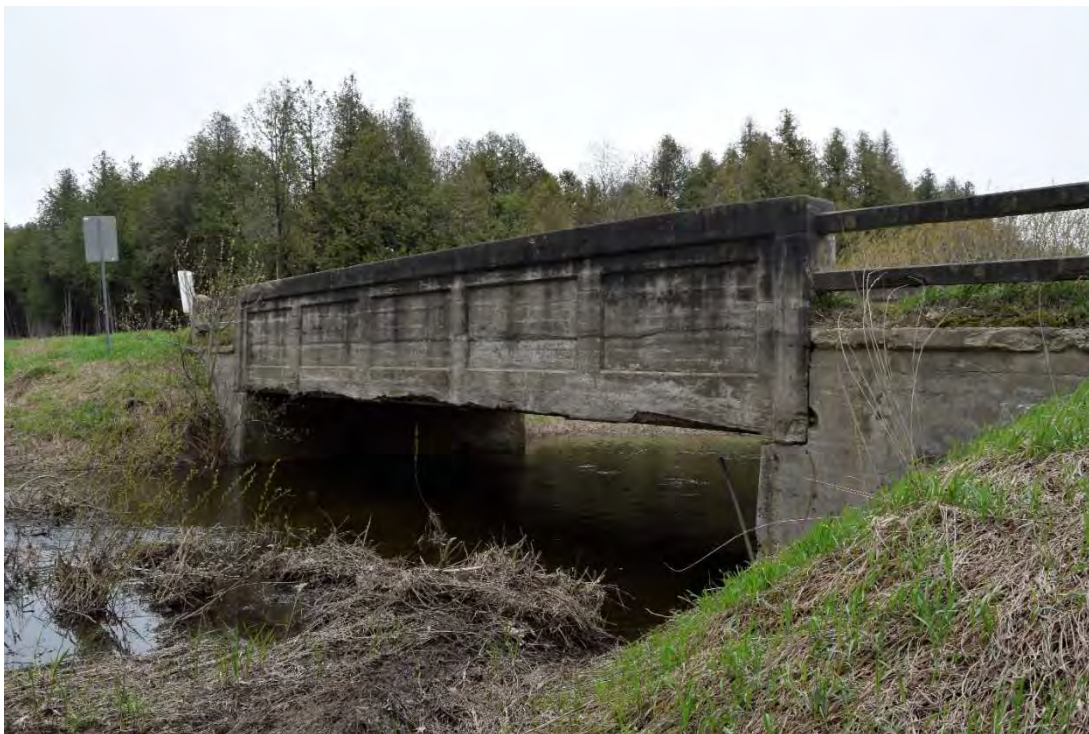
FIGURE 2: BRIDGE 2-WG, NORTH FACE, FACING SOUTH
