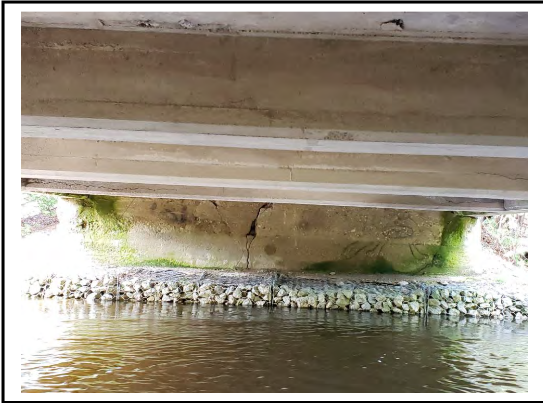
Photo 9 Underside of structure
