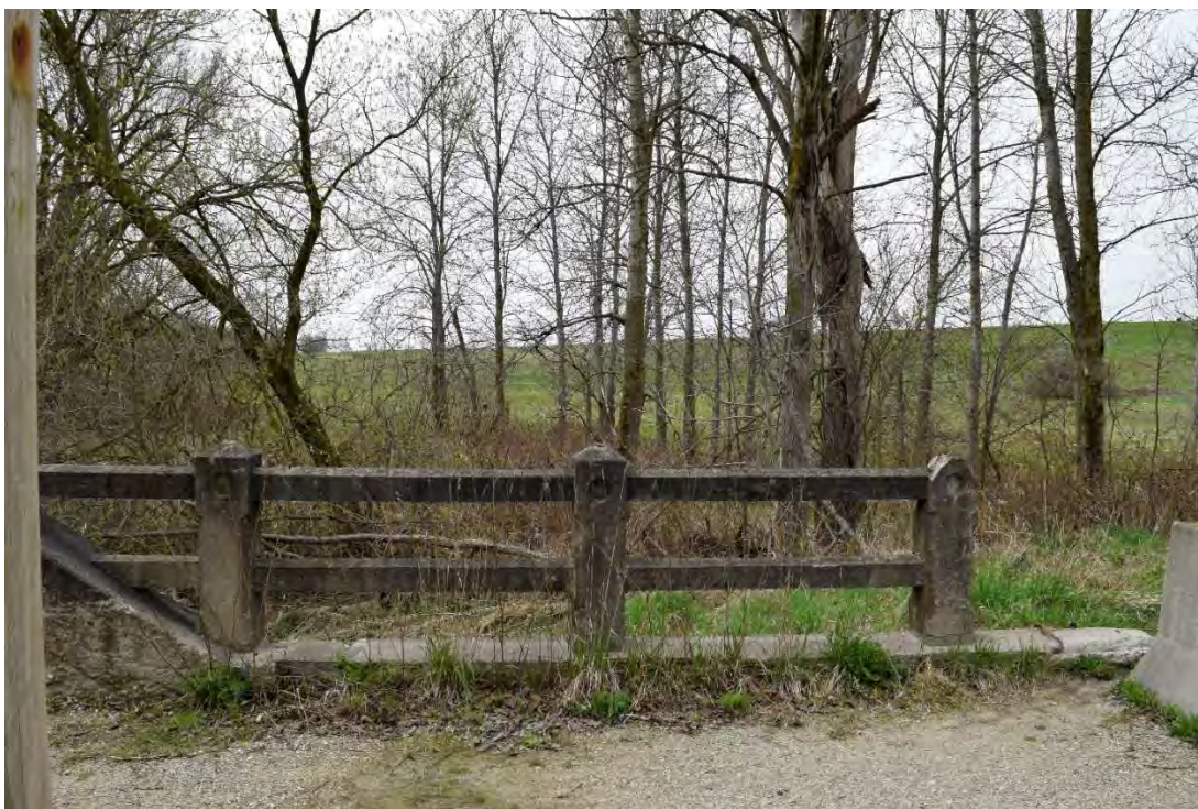
FIGURE 13: BRIDGE 3-E, TYPICAL GUARDRAIL, SOUTH SIDE
