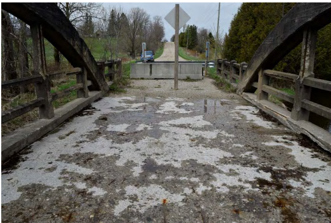
FIGURE 15: BRIDGE 3-E, BRIDGE DECK, FACING NORTHWEST
