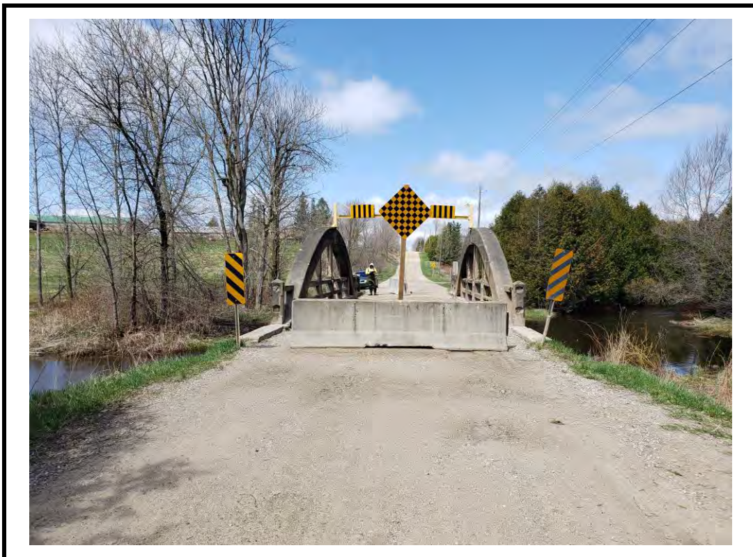
Photo 2 Structure from south approach
