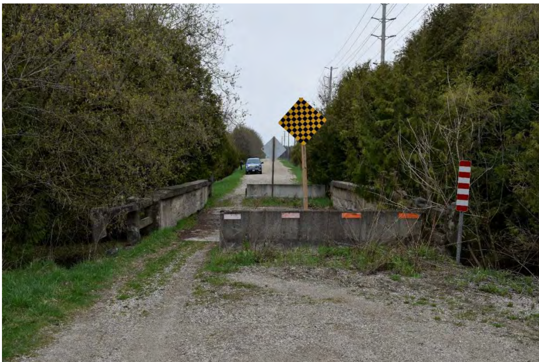
FIGURE 19: BRIDGE 5-E, LOOKING NORTHWEST FROM APPROACH
