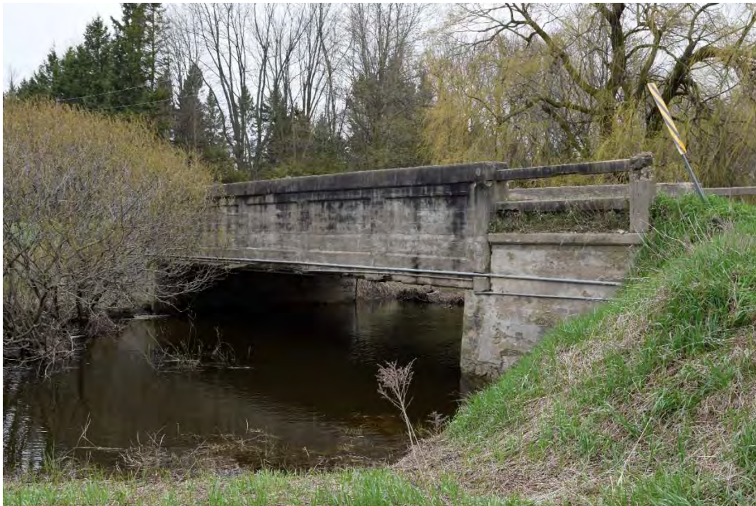
FIGURE 1: BRIDGE 2-WG, SOUTH SIDE FACING NORTH
