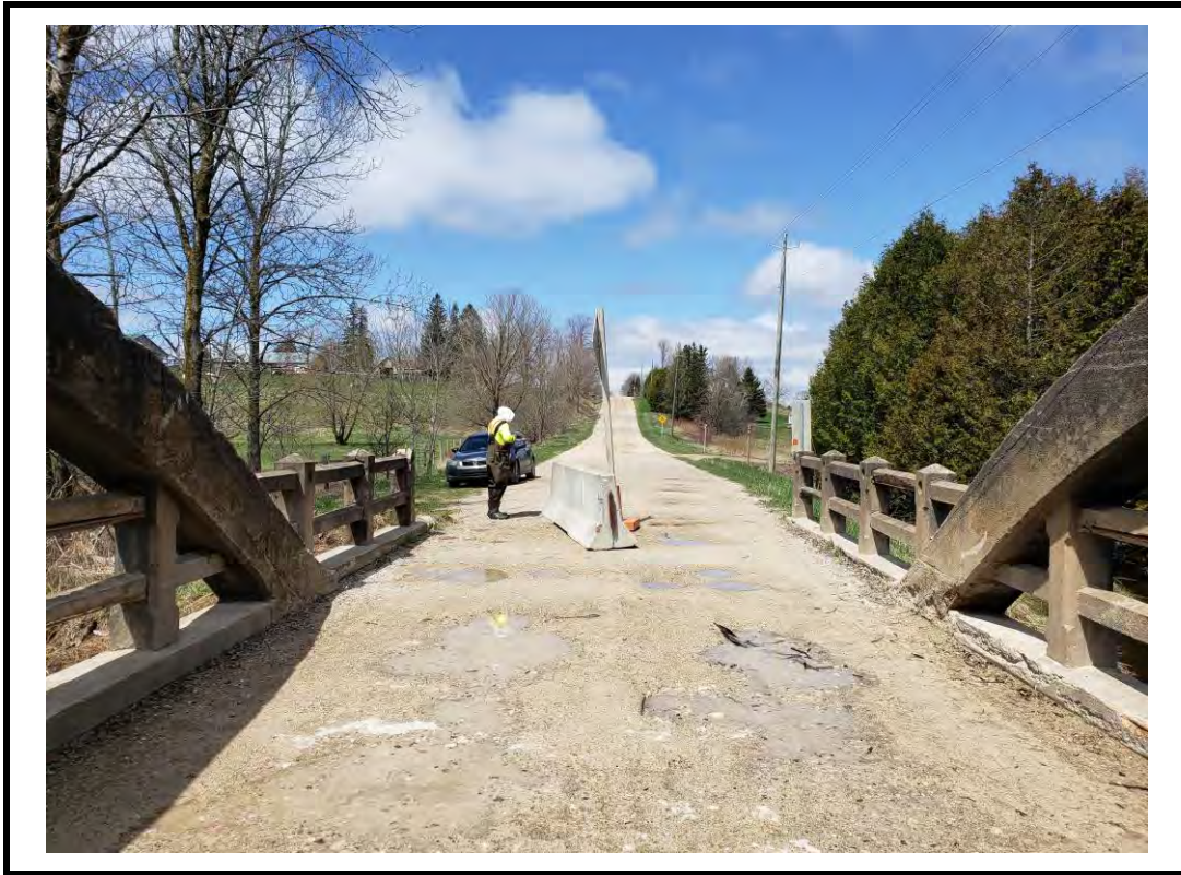
Photo 3 North approach from centre of structure
