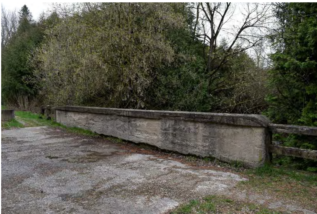
FIGURE 22: WEST SIDE OF BRIDGE 5-E WITH ROAD DECK
