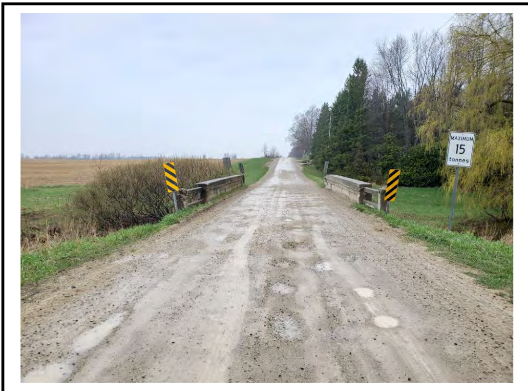
Photo 2 Structure from south approach
