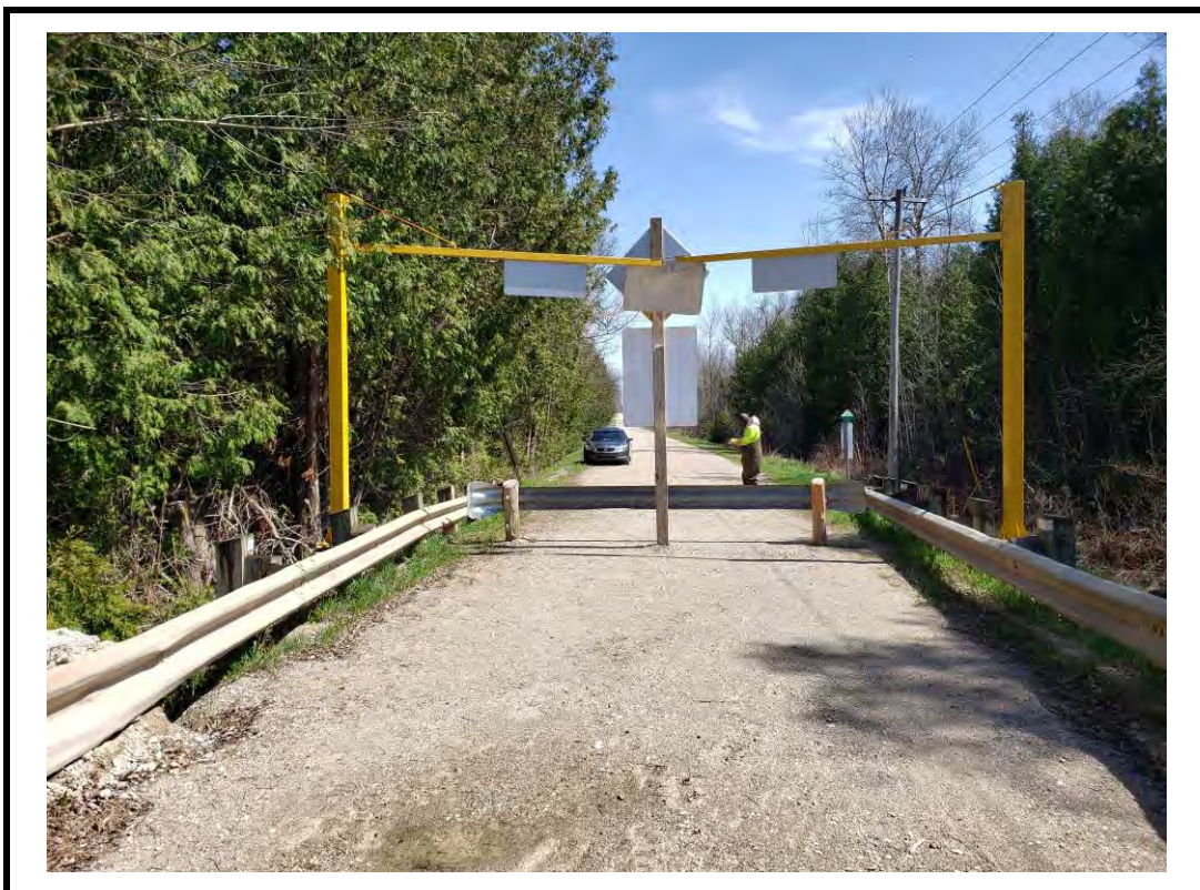
Photo 4 South approach from centre of structure
