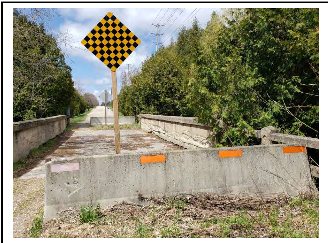
Photo 2 Structure from south approach
