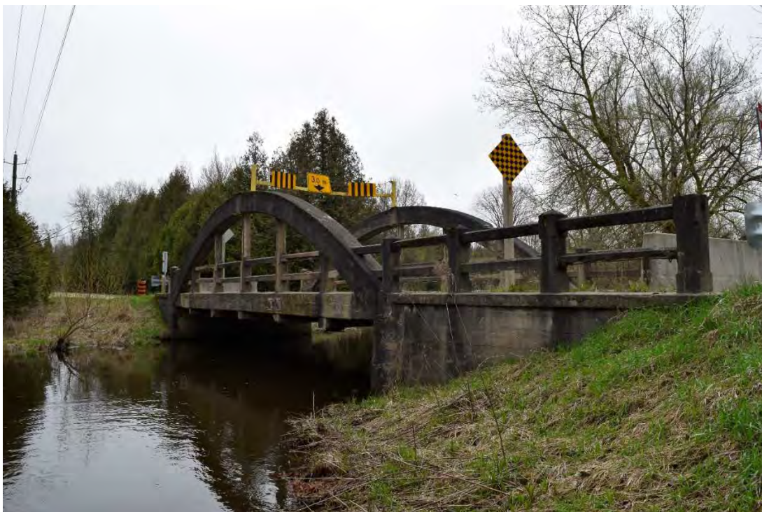
FIGURE 12: BRIDGE 3-E, SOUTHSIDE OF BRIDGE, FACING NORTH
