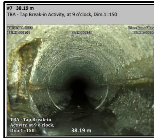
Victoria Crescent Sanitary Sewer
