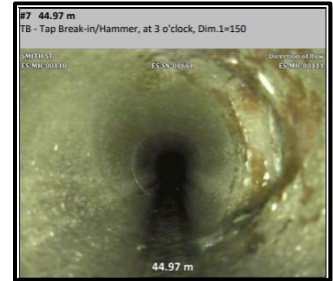
Smith Street Sanitary Sewer
